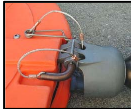
Properly Closed Gate Figure 11
